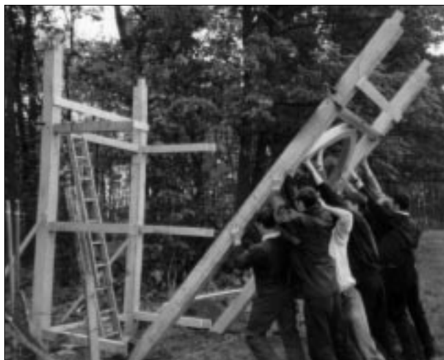
Above left: Work under way on the timber frame shelter roof during the show. Above right: Framework of lych gate under construction in workshop. Below left: Framework being lifted into position prior to show. Below right: Completed lych gate;
