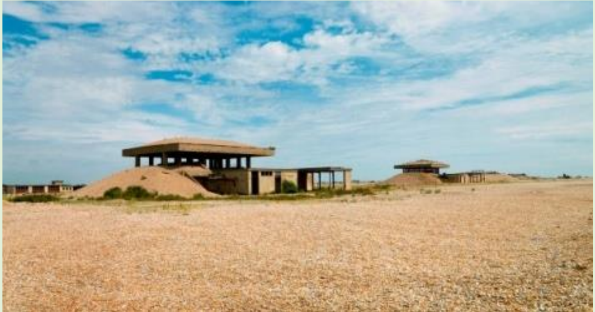
Cold War Installation, Orford Ness
