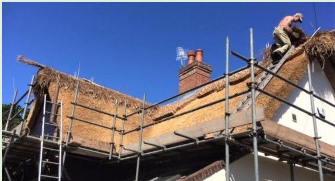
Thatching in progress © Barry Bridgwood
