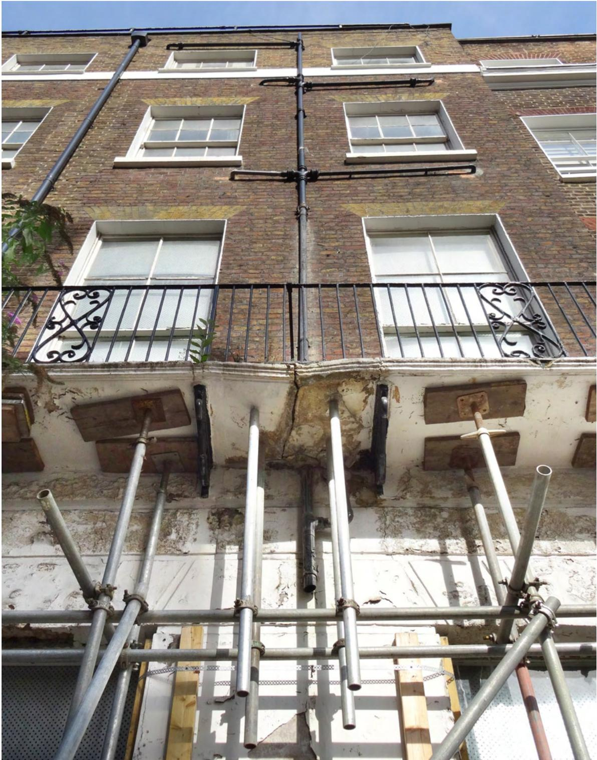
The consequences of a defective external drainpipe, London © Ingal Maxwell
