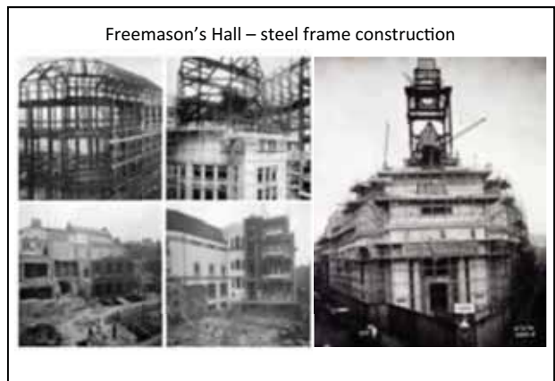
Freemason's Hall – Steel frame + Opening Ceremony June 1927
