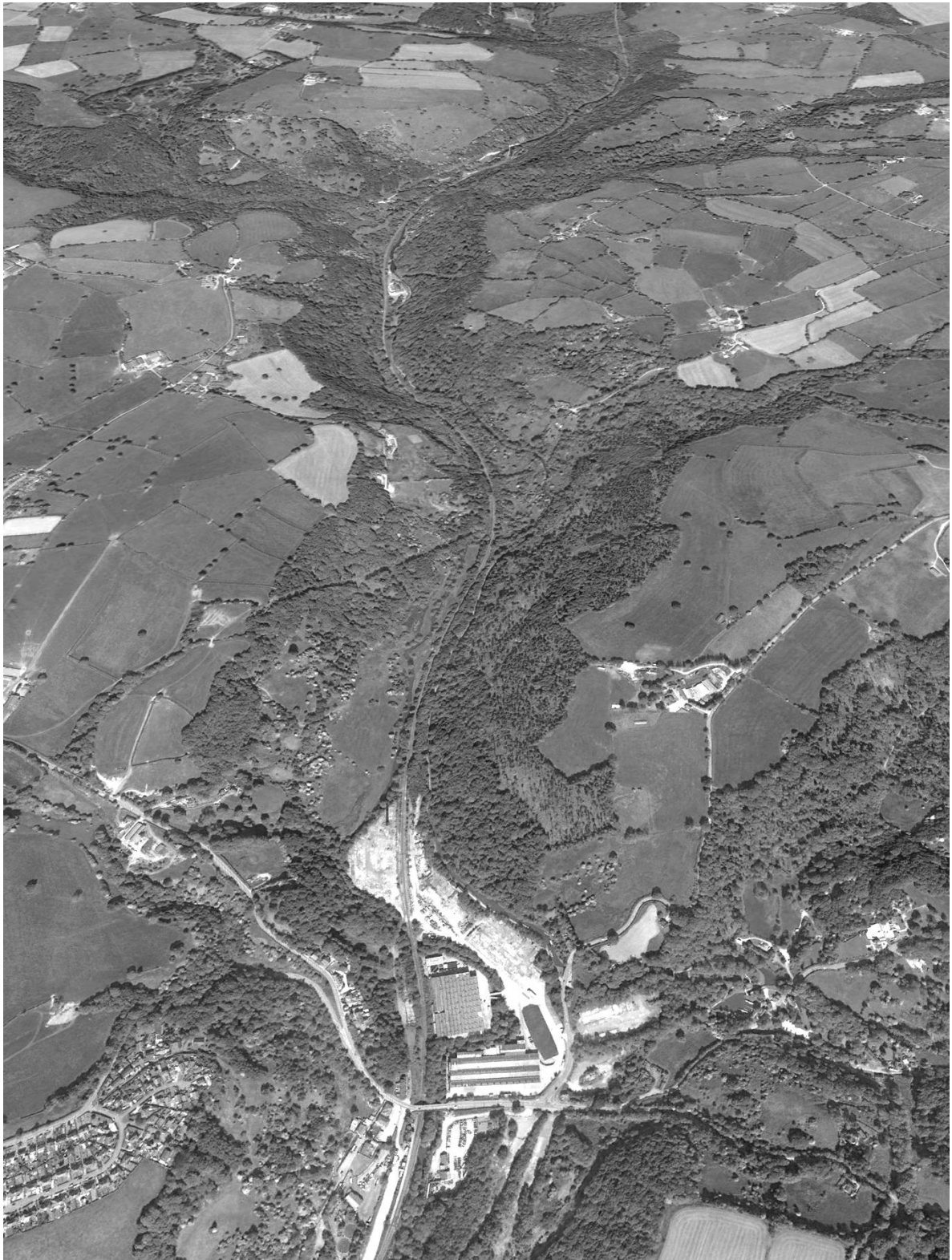
Fig.5.11 View to the north-west from the partially cleared Froghall industrial complex, and clearly indicating the winding route of the Churnet Valley Railway and Caldton Canal following the contours and meanders of the River Churnet valley floor. Image © Google Earth 2017
