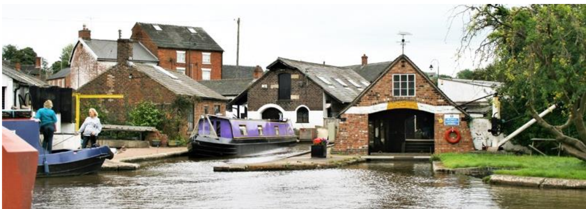
Fig.3.20 Trent & Mersey Canal narrow boat repair yard, Stone *
