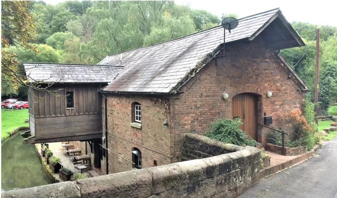
Fig.2.10 Former Caldon Canal Wharf Building given a new use as a tea rooms and cafe, providing refreshments for canal walkers and tourists at Froghall *
