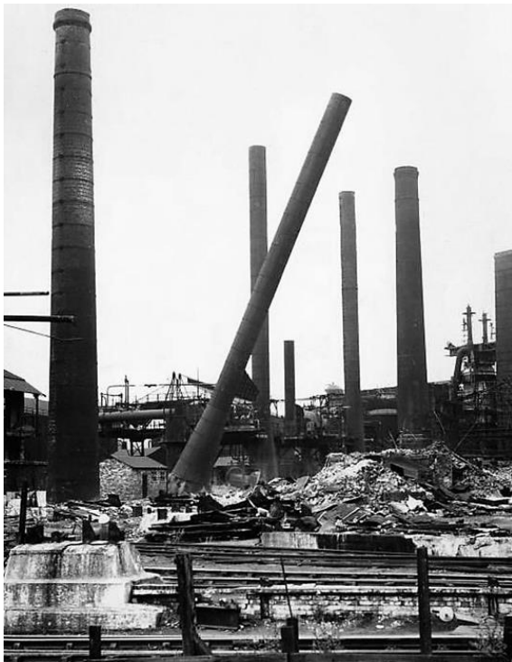
Fig.4.3 Chimney in process of demolition, Shelton Bar Steelworks. Image courtesy of The Potteries Museum & Art Gallery, Stoke-on-Trent
