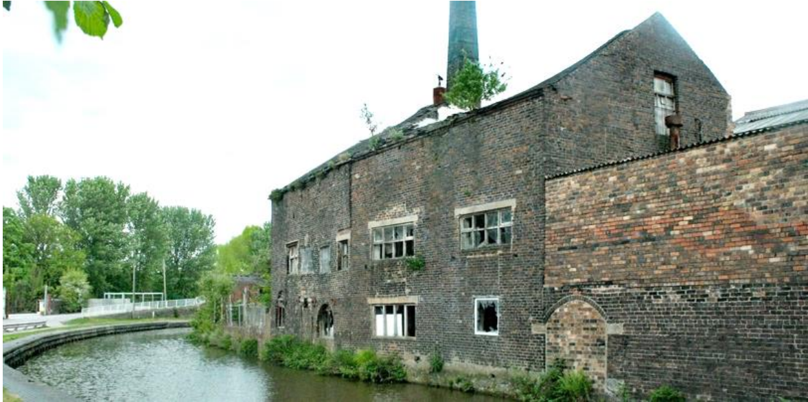
Fig.2.13 Advanced state of decline and decay of former Price's Teapot Factory at Longport on the Trent & Mersey Canal *
