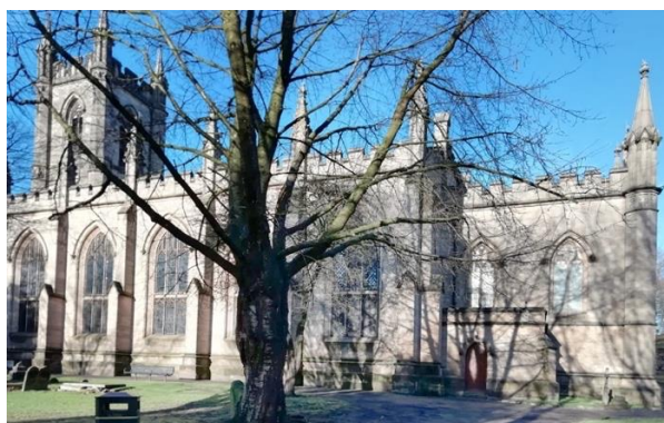
Fig.2.8 LHS: St Peter's Church, Stoke 1830 exterior * use. Image: Bethesda archive
