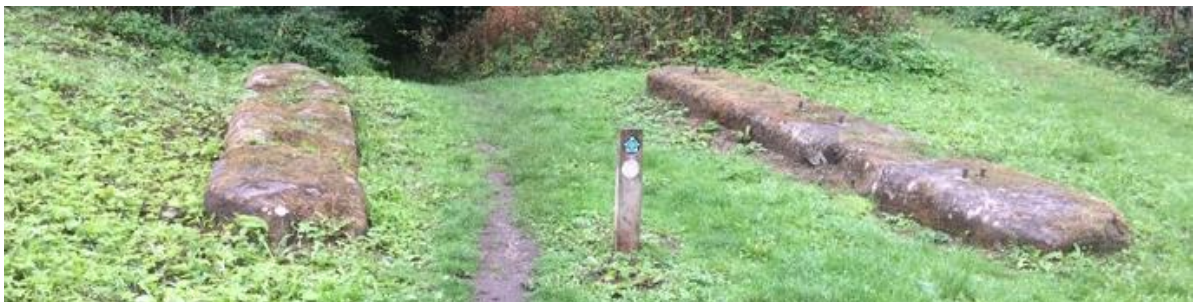
Fig.2.14 Tramway foundation base illustrating tangible remains *
