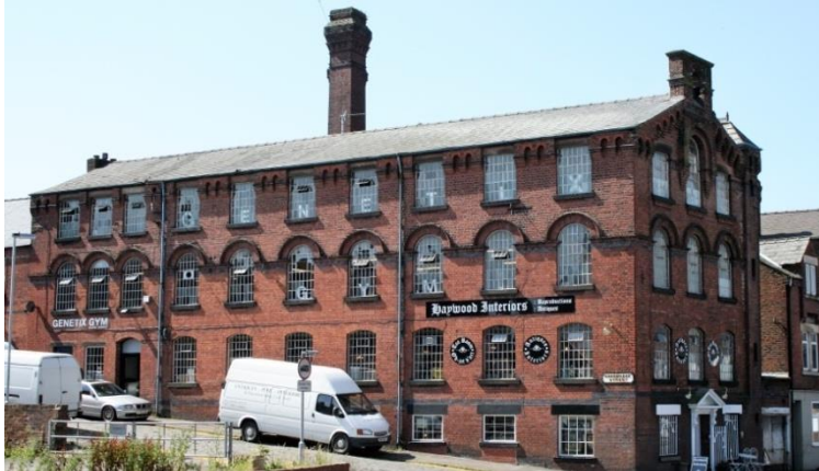
Fig.5.3 A former Leek mill building now used as a bar and restaurant*
