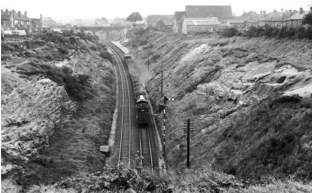
Fig.3.19 North Staffordshire Railway linking Derby and Stoke: Meir Station cutting.
