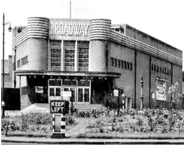
Fig.4.5 The Broadway Cinema 1936, Meir, subsequently demolished in 1973.
