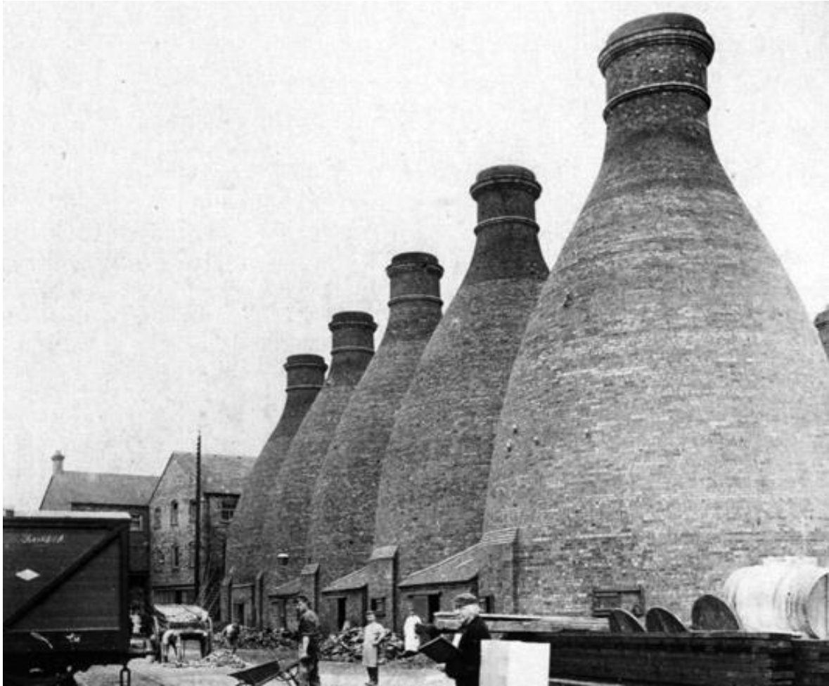
Fig.3.13 A bank of five unusually large brick hovel ovens at the Twyford's Cliffe Vale factory accommodated the firing of large sanitary ware products. Their complex structural shape is more easily created using bricks, requiring considerable brick-laying skills to accomplish with both the curved inner and outer faces inclined inwardly through progressive corbelling (or projecting) of each successive course over the next. Image © Warrillow Collection, Keele University Library (Warr 1045)
