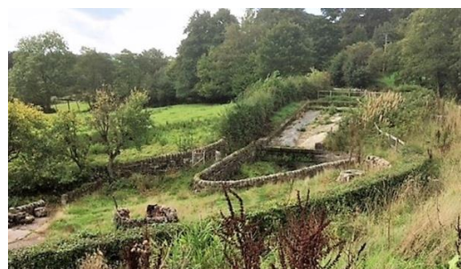
Fig.5.8 Leek Branch Canal weir overflow, sluice and drain near Longsdon *
