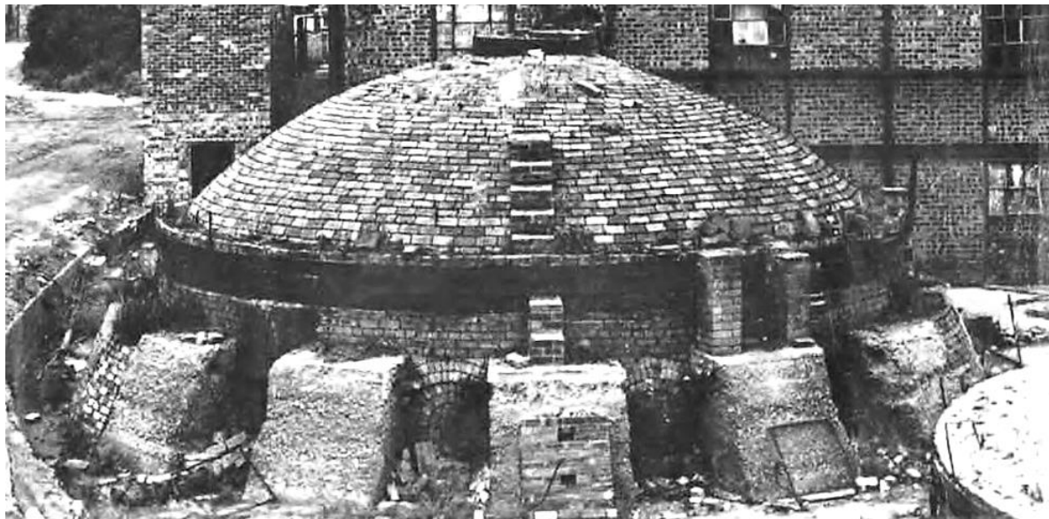
Fig.3.10 Typical brick Beehive Kiln with intermittent support buttressing to secure the dome structure in addition to the surrounding iron banding. Otherwise, the dome would be prone to collapse (See YouTube video clip at https://www.youtube.com/watch?v=SMA66ZDElqY for when the constraining iron band is cut through unthinkingly)
