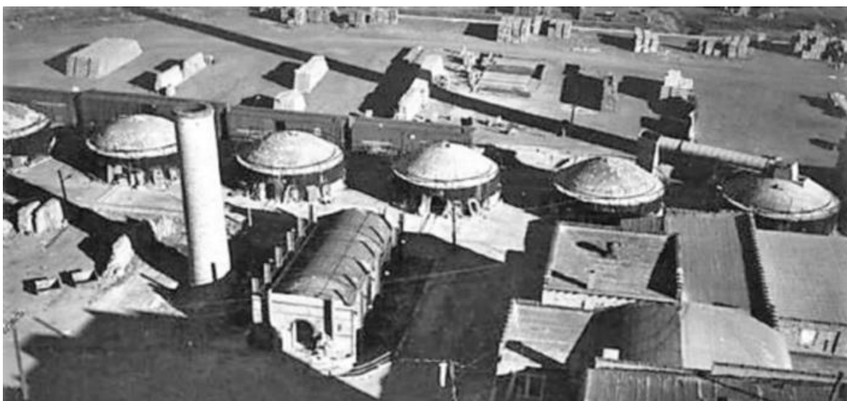
Fig.2.41 Aerial view of a brickworks showing 6 beehive kilns used in brick making, with a tunnel kiln and its smoke stack to the centre left
