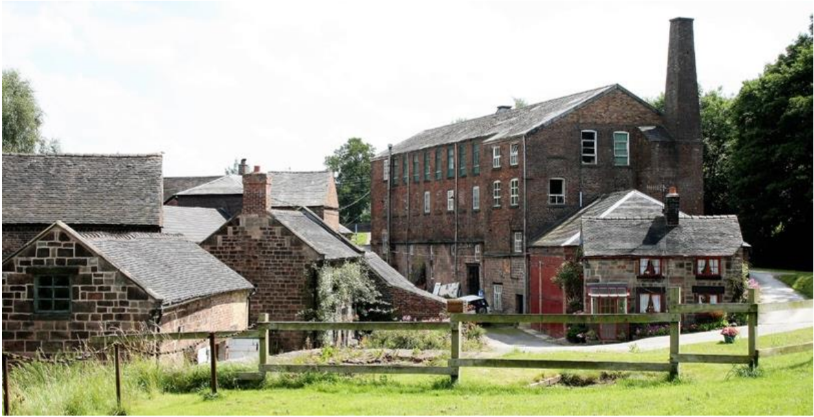
Fig.8.7 Cheddleton 4-storey flint processing mill and Overseer's Cottage *
