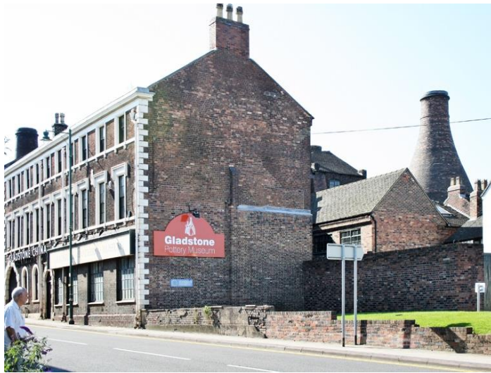
Fig.3.0 Gladstone Pottery Museum, Longton. The formal frontage has the factory courtyard and hovel oven to the rear *
