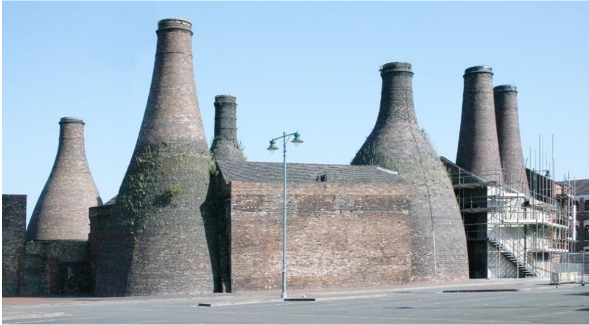
Fig.8.5 The Gladstone Pottery Museum range of buildings. Saved from demolition in 1971 it has been restored and is now operating as a pottery processes museum and information centre in Longton *
