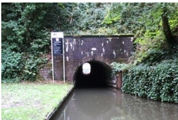
Fig.2.4 Froghall tunnel's limited headroom *
