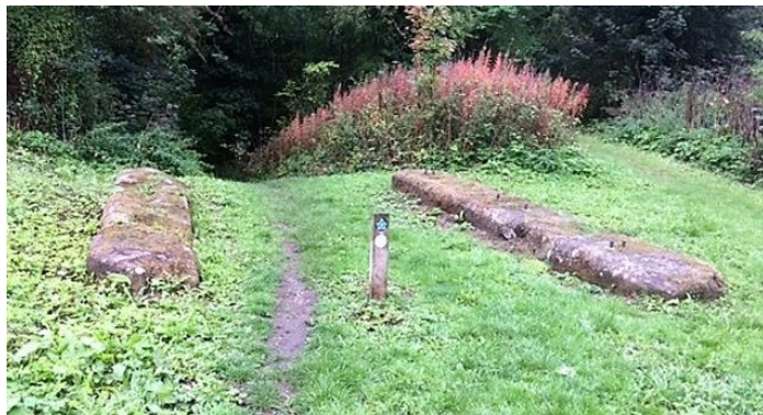
Fig.2.12 Cable tramway braking system foundations above the lime kilns at Froghall at the top of an incline down to the wharf level *
