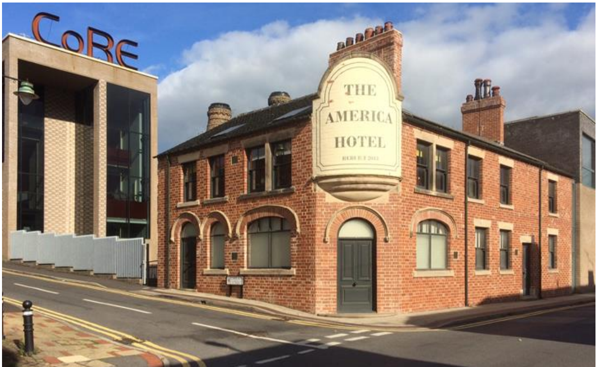
Fig.9.5 A CoRE scheme after repair and restoration work, Normacot. Originally, the pub was called The American, not the America Hotel *
