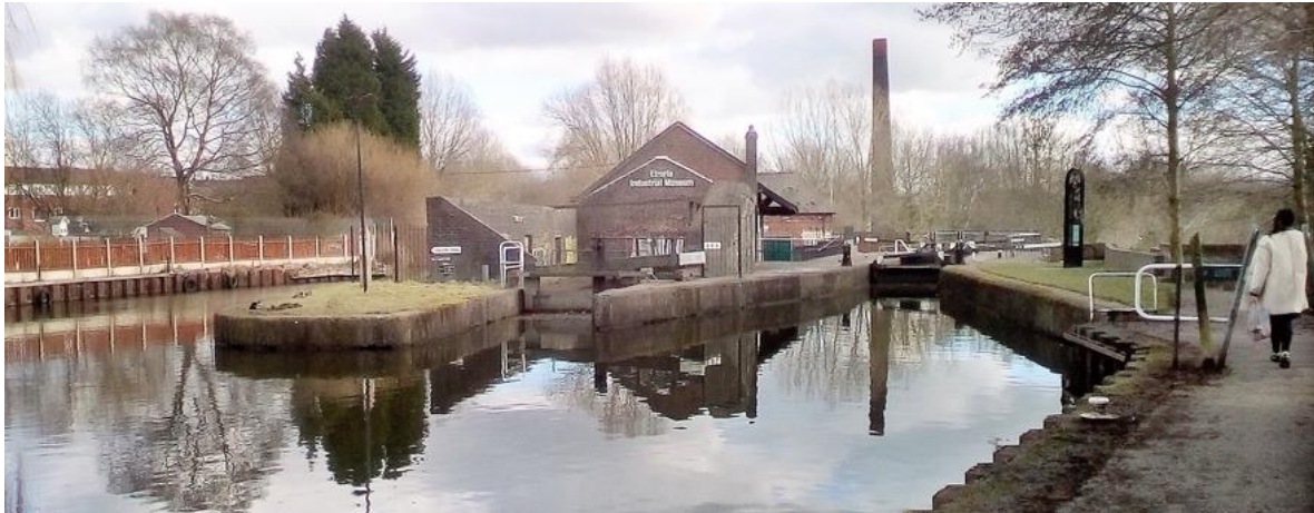
Fig.8.10 Caldon Canal (on the left) brought materials from its upper reaches to Etruria for processing. The Trent & Mersey was used for distribution to the various factories. The summit lock connecting the two canals were particularly deep, with a total drop of some 20 feet (6m) *
