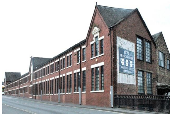
Fig.4.14 Long formal front of the Emma Bridgewater Factory, Lichfield Street, Hanley * See also Fig.3.8 for an aerial view from 1934
