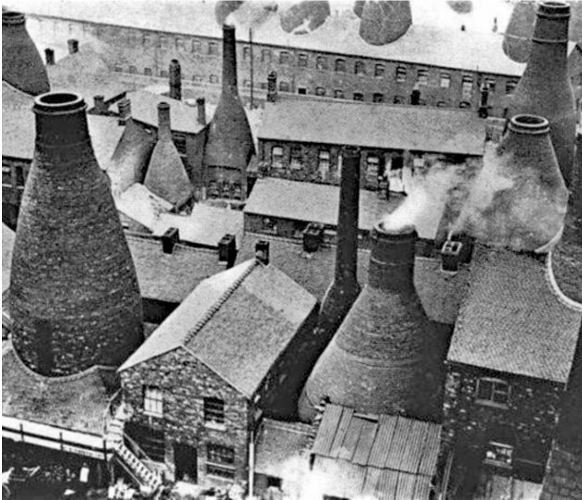
Fig.6.0 Typical courtyard clutter of buildings as factories developed and expanded with at least four different types of ovens/kilns and a more formal external street frontage
