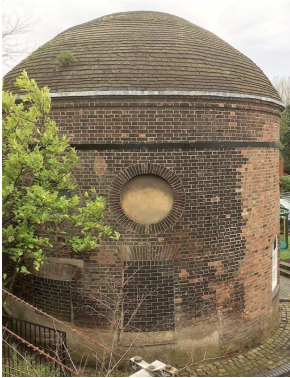
Fig.3.5 The remains of the original Wedgwood Etruria Factory Roundhouse *
