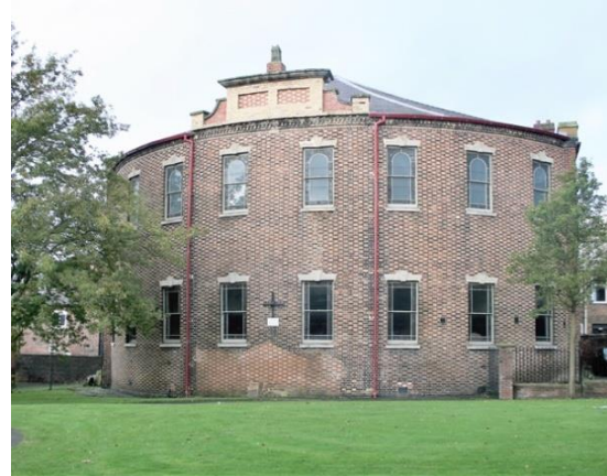
Fig.4.11 Bethesda Chapel rear Apse of Flemish bond brickwork *
