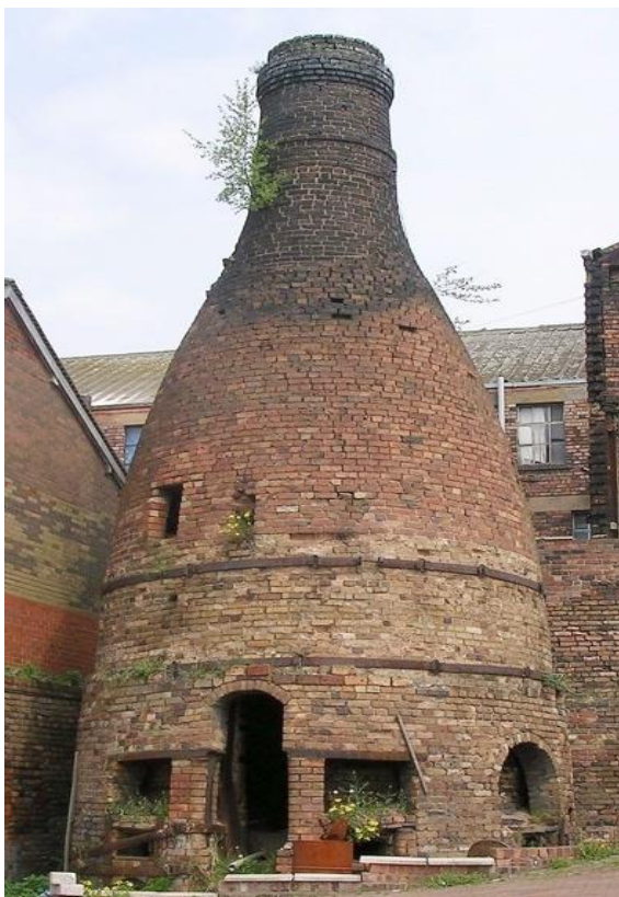
Fig.2.34 Updraught skeleton bottle oven with external reinforcing Bonts Image courtesy Phil Rowley
