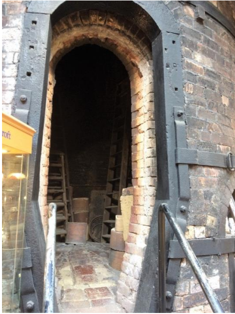
Fig.2.30 Inside an inner firing chamber with saggars stacked ready for firing. The inner chamber of updraught and downdraught kilns had domed floors over the underlying flues. External horizontal iron bands or Bonts reinforced the inner chamber to cope with high temperature variations during firing and cooling *
