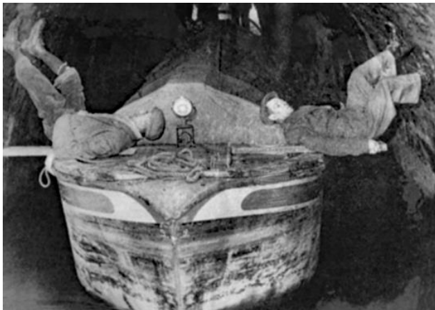
Fig.2.1 Legging it through Harecastle tunnel on the Trent & Mersey canal. Image: A.H. Body
