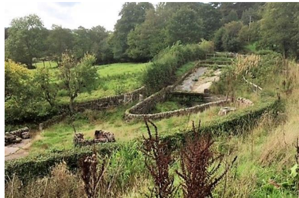
Fig.2.6 Leek Branch weir overflow, sluice and drain near Longsdon *
