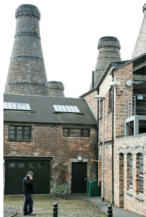
Fig.9.3 Former Enson pottery hovel ovens, now the CoRE Centre, Normacot *
