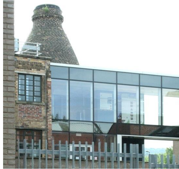
Fig.1.4 Refurbish and new-build work at the CoRE Centre (formerly Enson Pottery), Normacot *
