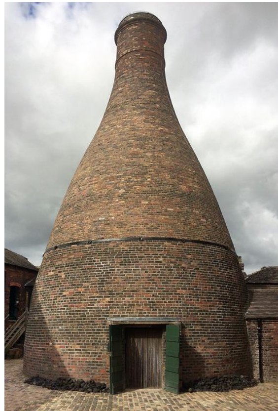
Fig.2.32 Oven hovel external view displaying the relevance of using bricks for the construction to create the complex bottle shape, Gladstone Pottery Museum *
