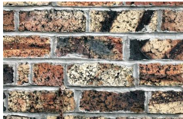
Fig.2.43 Typical appearance of local brickwork. Probably, Longton Hall bricks *
