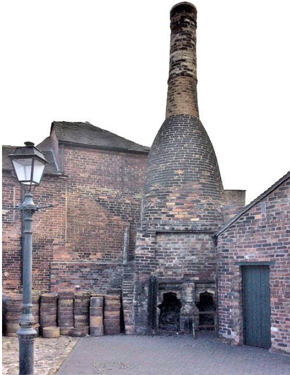
Fig.2.22 A typical muffle kiln used during firing of decorated ware, Gladstone Pottery Museum *
