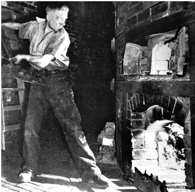
Fig.2.26 The limited space between hovel and firing chamber © Wedgwood Archive, V&A
