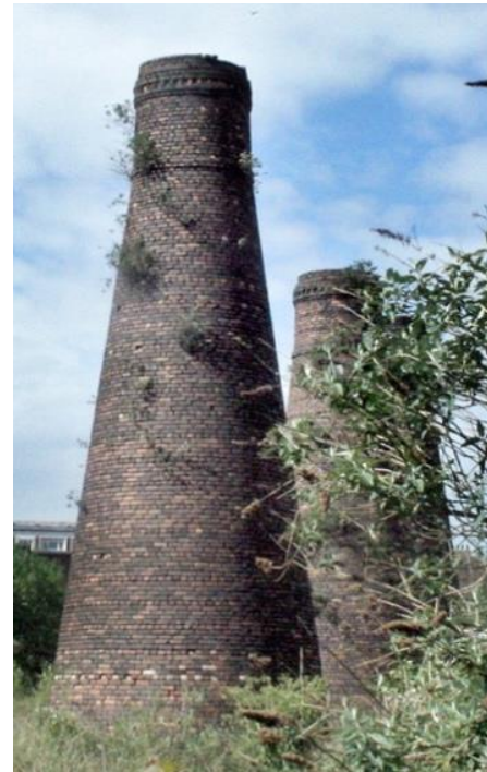
Fig.2.21 Three Listed downdraught ovens, part of the demolished Acme Marls factory, Bournes Bank, Burslem *
