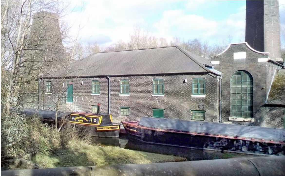
Fig.8.12 Shirley's Mill square-plan calcining kiln, upper-level tub grinders floor, ground floor drive shafts and steam powered beam engine housing with exhaust chimney *
