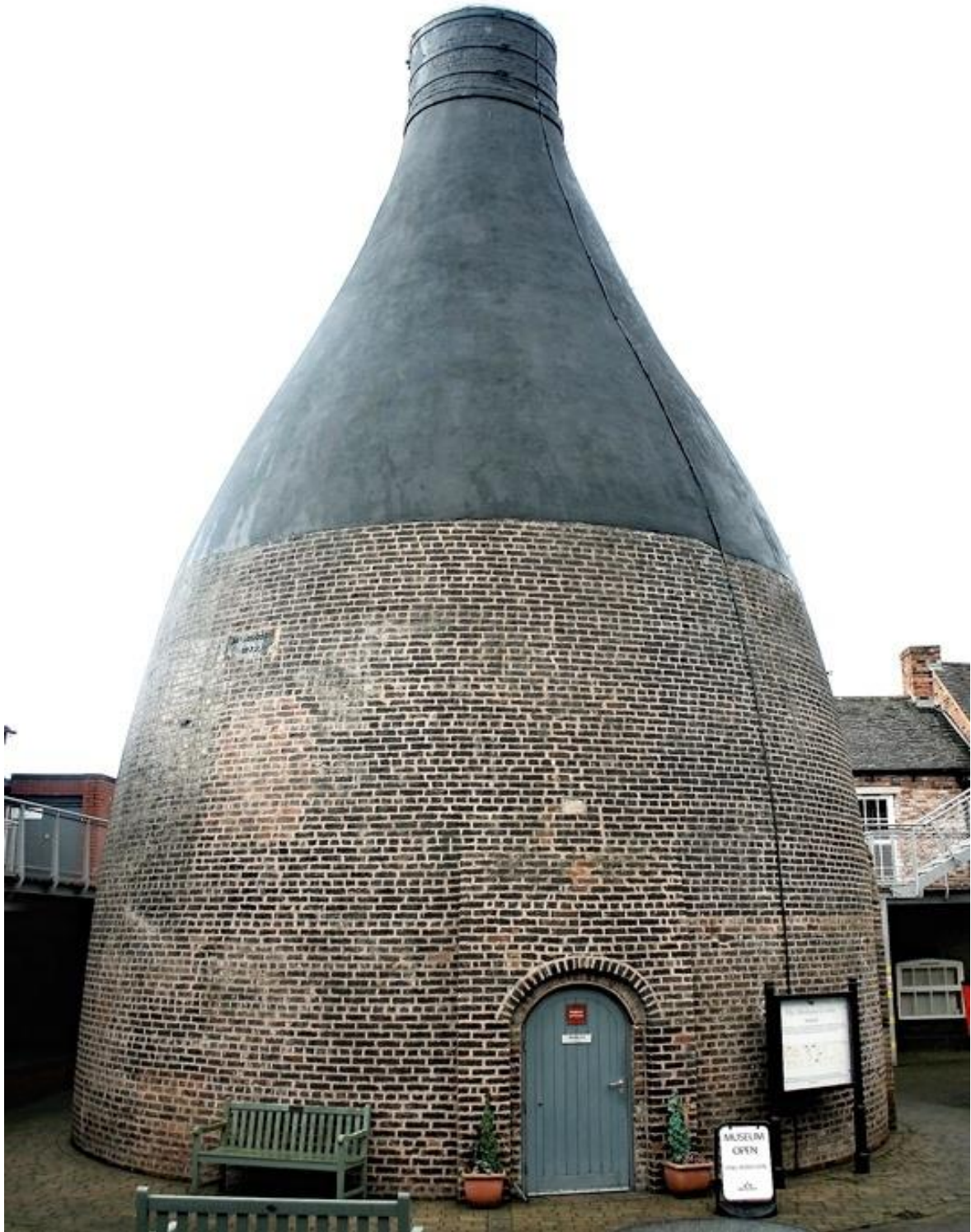
Fig.8.21 Dudson Centre restored courtyard bottle hovel. A plaque records 1872 as the construction date *
