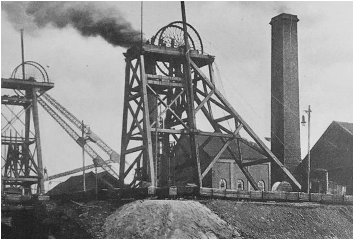
Fig.2.18 Typical early pit-head winding gear Glebe Colliery, Fenton (closed 1964). Image courtesy of The Potteries Museum & Art Gallery, Stoke-on-Trent
