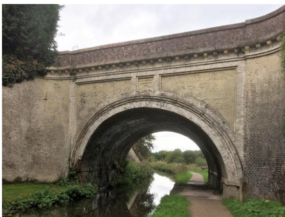
Fig.2.7 1841 Hazelhurst Aqueduct, Caldon Canal below with Leek Branch above *
