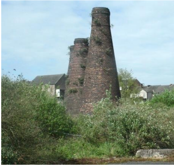
Fig.1.3 Abandoned bottle ovens at Bournes Bank, Burslem *
