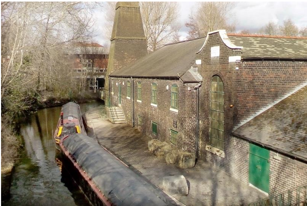
Fig.8.11 The lower Trent & Mersey canal level at Etruria (Shirley's Mill) with a square-plan calcining kiln at the end of the main building. The beam engine is behind the large round-headed window and tub grinders are on the windowed upper floor *
