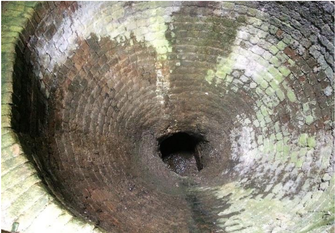
Fig.8.14 Shirley's Mill calcining kiln well in unfilled state *
