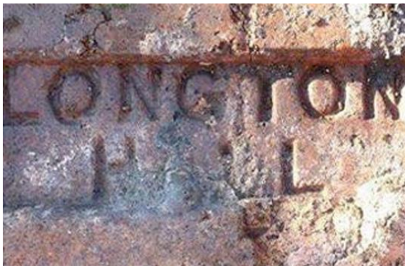
Fig.2.42 Typical stamped brick frog from the Longton Hall Brickworks *
