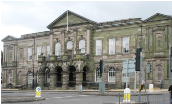
Fig.4.3 Longton Town Hall and market hall (Recently cleaned and going green) *
