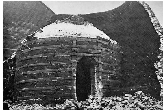
Fig.2.33 Updraught inner firing chamber showing reinforcing iron bonts , and the partly demolished hovel surrounding the inner structure at the Copeland factory (1960) Image source unknown
