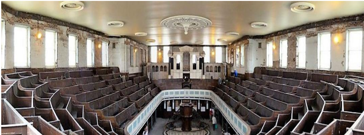
Fig.4.12 Bethesda Chapel interior after Phase I repair and restoration work. Image: Bethesda Archive
