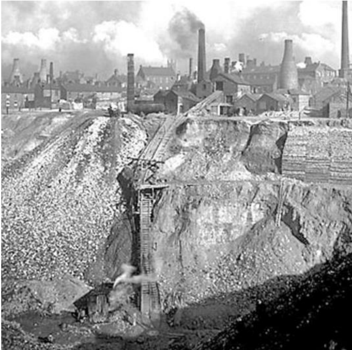
Fig.4.0 Daisy Bank brickworks marl hole Longton, c1900. This open cast mine supplied clay for its adjacent brick and tile works showing the central image track for transporting the clay directly into the works above the pit. To the left, pottery waste or shraff is being tipped as backfill. The site has since been completely backfilled and built over as a small industrial estate. Shraff tips were also locally known as shard rucks . William Blake Image courtesy of The Potteries Museum & Art Gallery, Stoke-on-Trent
