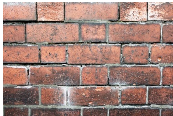
Fig.2.45 Semi-glazed brickwork resulting from higher firing temperatures are more resilient *
